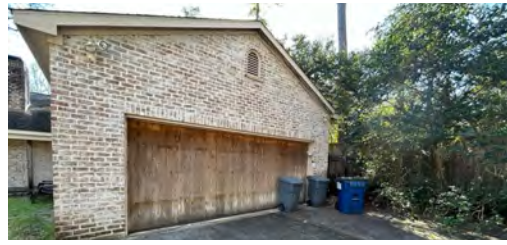
garage door water damage
