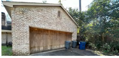
garage door water damage
