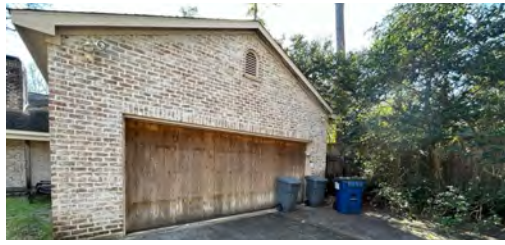
garage door water damage
