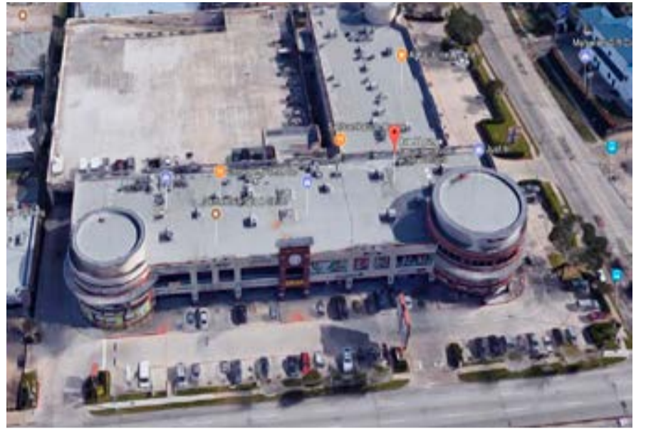
Avani Lounge, Harris County 5711 Hillcroft Suite D6, Houston Violation date: April 27, 2017
